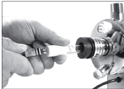
Step 4 & 5 - Remove Sockets
